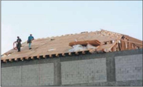
Construction loads are those loads imposed on the unfinished building as a result of the construction process. Typical construction loads include the weight of the workers, equipment, and building materials, to name a few. For example, a bundle of plywood or gypsum board stacked on trusses temporarily creates construction loads.
